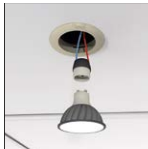
3. Connect the bulb to the socket and lock into the correct position.
