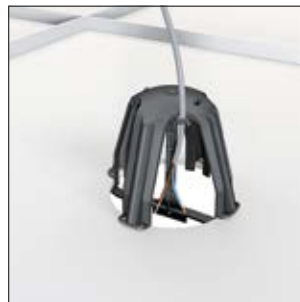
2. Push the spikes into the plasterboard to prevent shifting and disconnect the tool.
